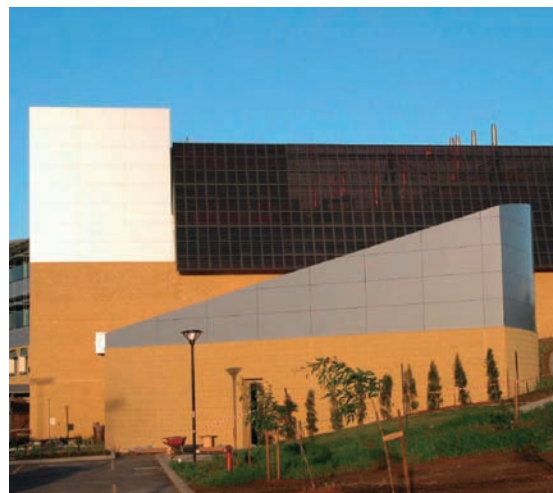
Figure 11. Dye-sensitized solar glass panels integrated in the wall of the CSIRO research building in New Castle, Australia.
